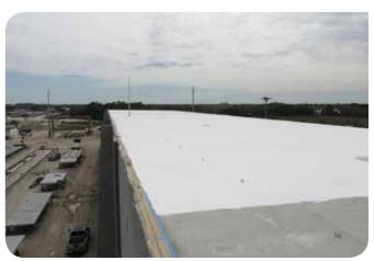
Over the course of three weeks, the crew members finished the system. They pressure-washed the roof and then spray-applied two passes of the WeatherBloc-IC to achieve an average dry film thickness of 20 mils (508 microns).
