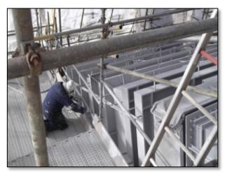
A New Zealand based operations company utilized ducting systems within many areas of their facility. During operation these ducts vibrated as hot air passes through them causing noisy conditions for employees and impacted on site noise requirements. A Mascoat Specialist conducted an assessment of the ducting and recommended using Mascoat's sound dampening coating. This coating was then applied to the ducting at a thickness of approximately 2.5 mm (5 coats of 0.5 mm each).
