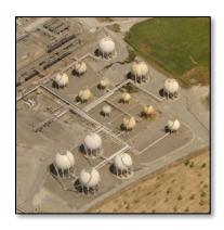
In 2009, two different facilities used Mascoat Industrial-DTI on a total of three LPG spheres. These spheres were dealing with radiant heat gain/solar loading issues. These issues would increase the amount of Liquefied Petroleum Gas (LPG) that vented to the flare header.
