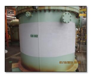
Phosgene (CoCl<sub>2</sub>) is an extremely hazardous, odorless gas, dangerous enough to use as a chemical weapon during World War I. A chemical plant in Baytown, TX was concerned about CUI on their Phosgene tanks and risking a resulting chemical release, so the facility left their tanks un-insulated for years.
