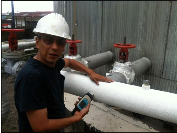
A test was setup to prove the performance of the coating. The pipe was already coated with an inorganic zinc, so there was no need to prime it. The chemical company wanted the surface temperature of the pipe to be below 176°F (80°C). The results of the test are as follows:
